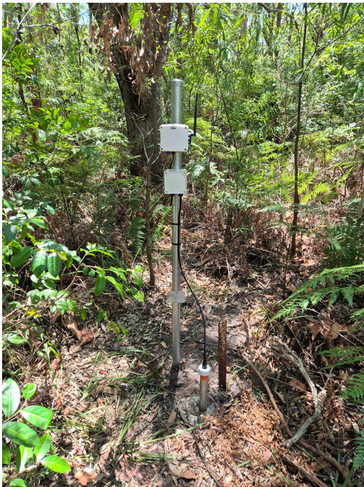
Plate 3 Live Monitoring Equipment installed at SK3520
