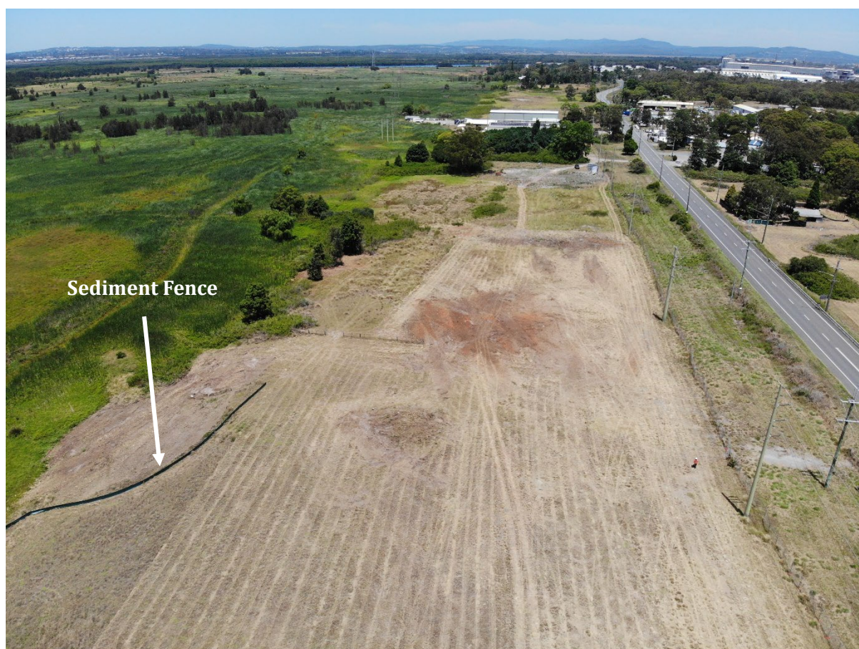
Plate 4 Sediment Fences Installed During the Reporting Period
