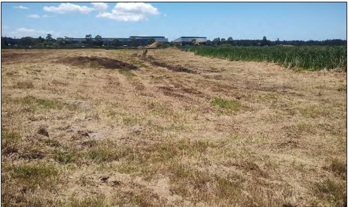
Figure 3: Cleared vegetation looking east (3/12/25). WesTrac site and Lot 210 fill stockpile in background. Low-lying parts of Lot 210 on right
