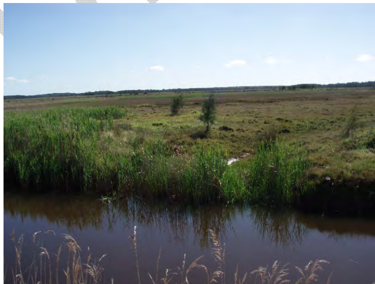
Photo 1 Overflow from Tomago North-South Drain into rehabilitated salt marsh
