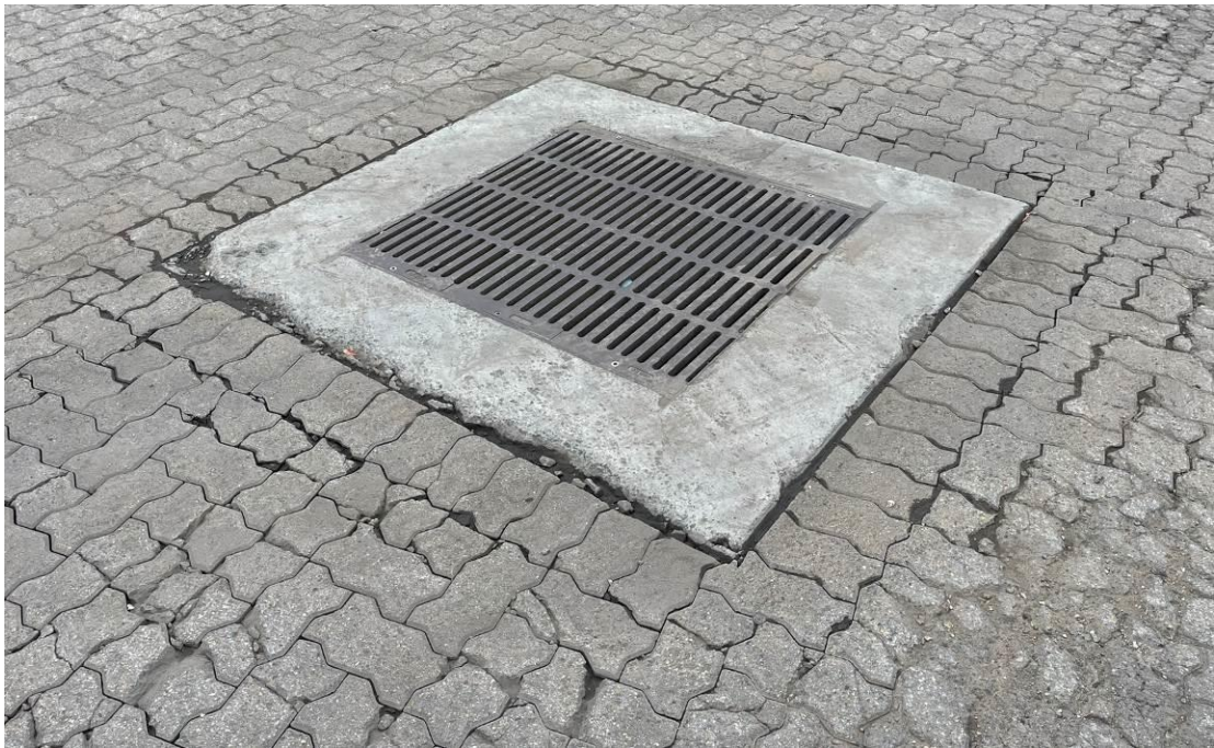
Photo 8: Drains within paved areas
