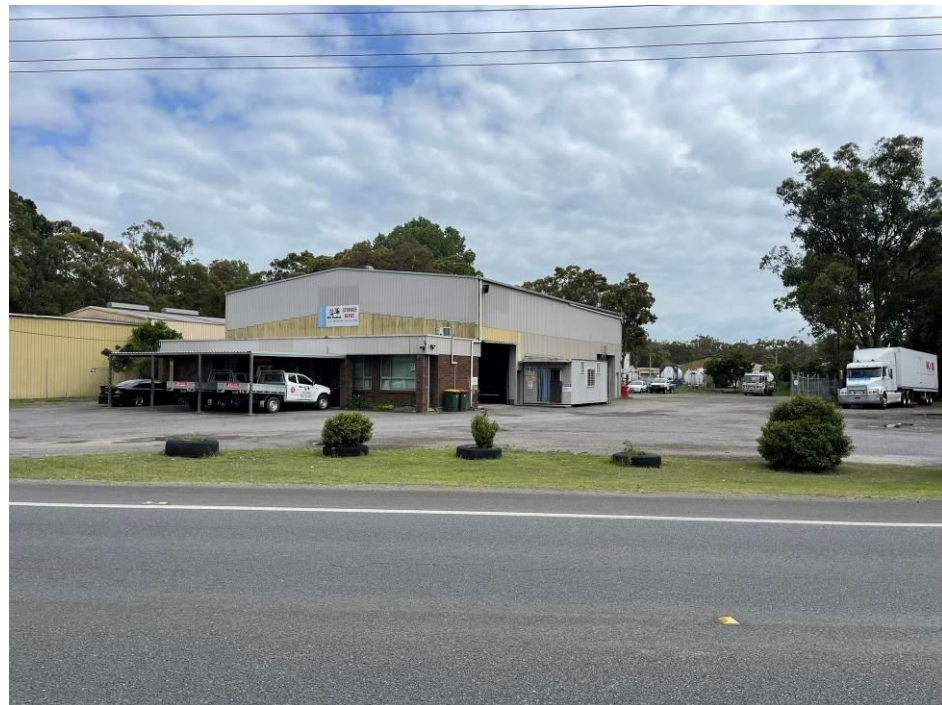
Photo 32: Industrial / commercial site north-west on Tomago Road
