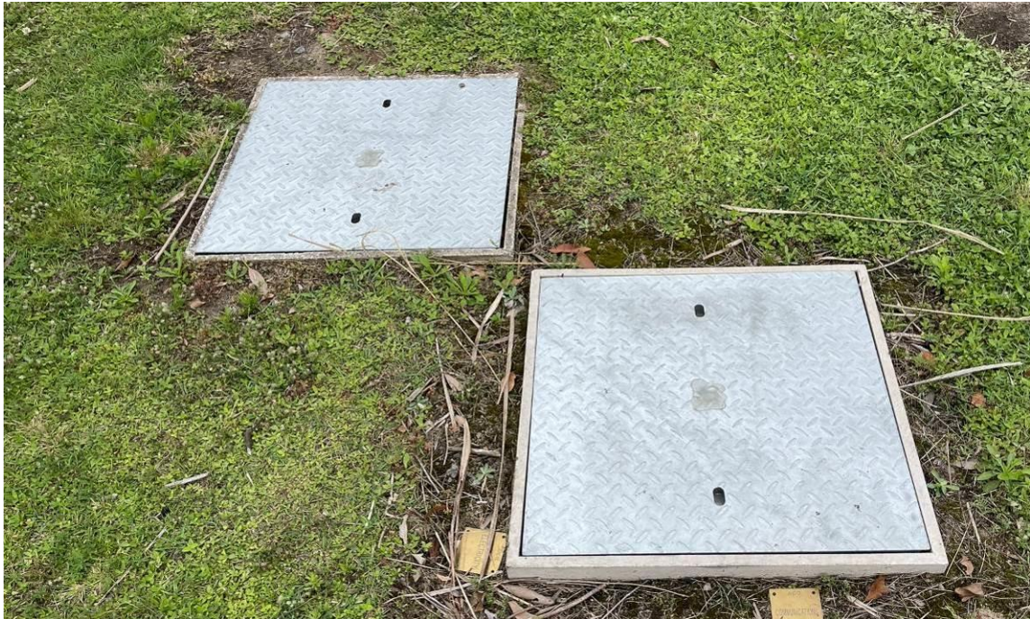
Photo 12: Service inspection pits
