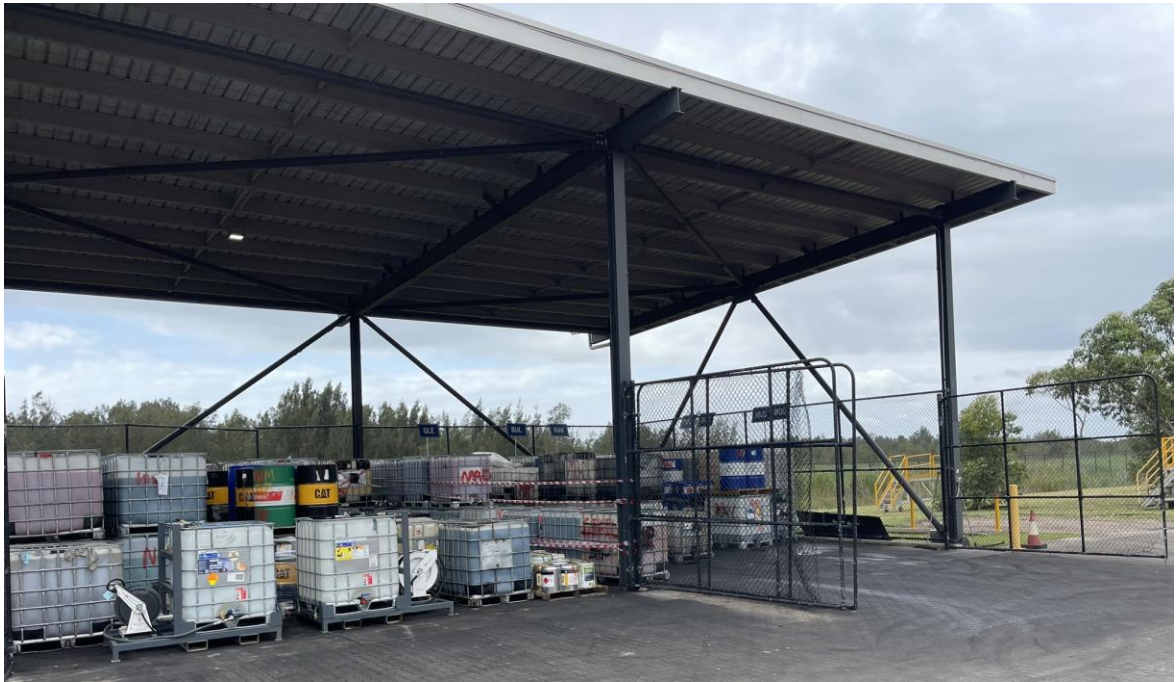
Photo 15: Bulk oil storage within bunded waste depot
