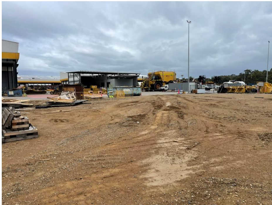
Photo 20: Hardstand areas in eastern parts of Stage 1
