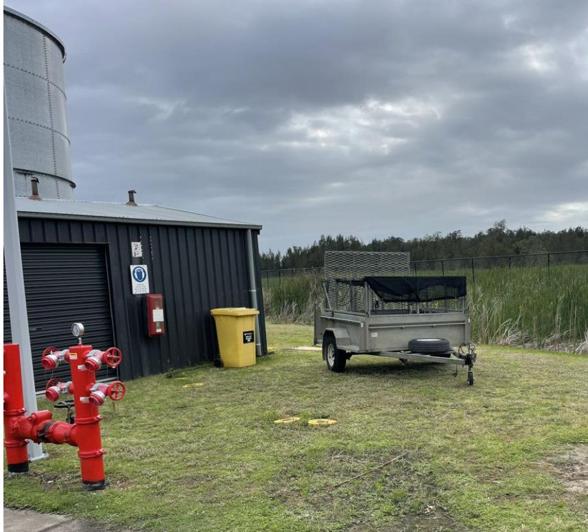
Photo 11: Water storage containers for fire suppressant. Southern swale in background
