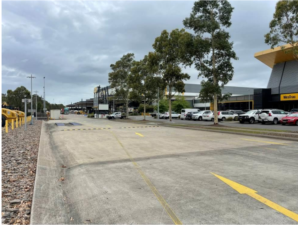
Photo 25: Internal concrete roads in the northern portion of the site
