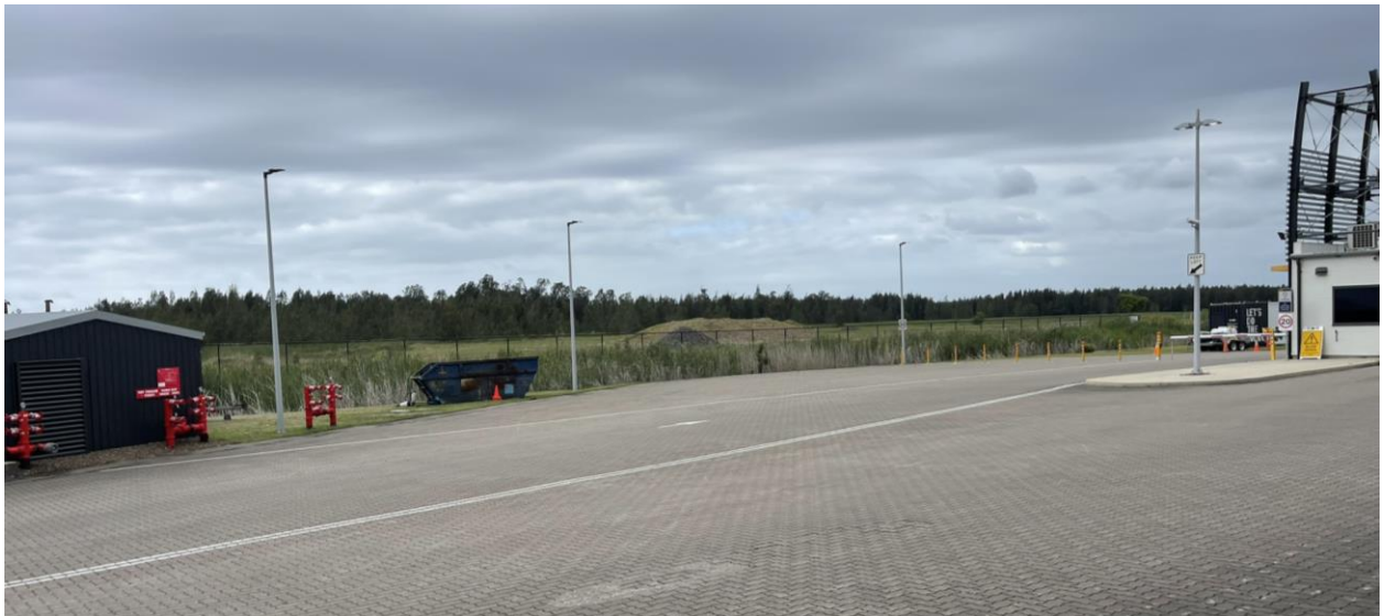
Photo 10: Paved areas in south-western corner near security office. Demonstration bay in background
