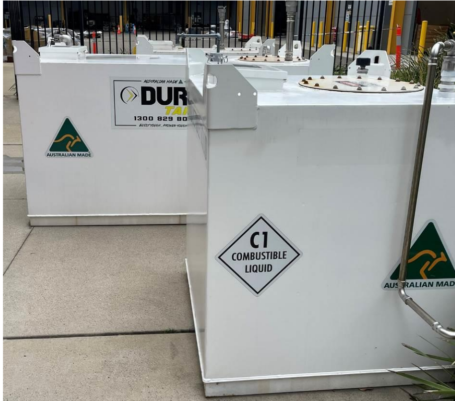
Photo 1: Self bunded coolant (1000 L)
